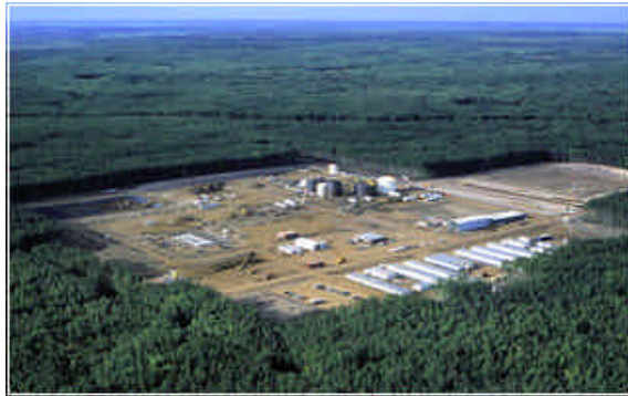
Construction of Mac Kay River (PetroCanada)
