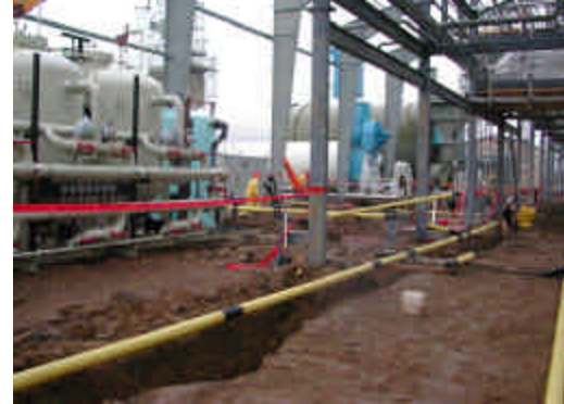
Construction of Christina Lake (EnCana)
